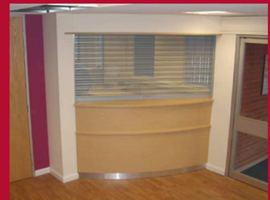
Security shutters fitted
